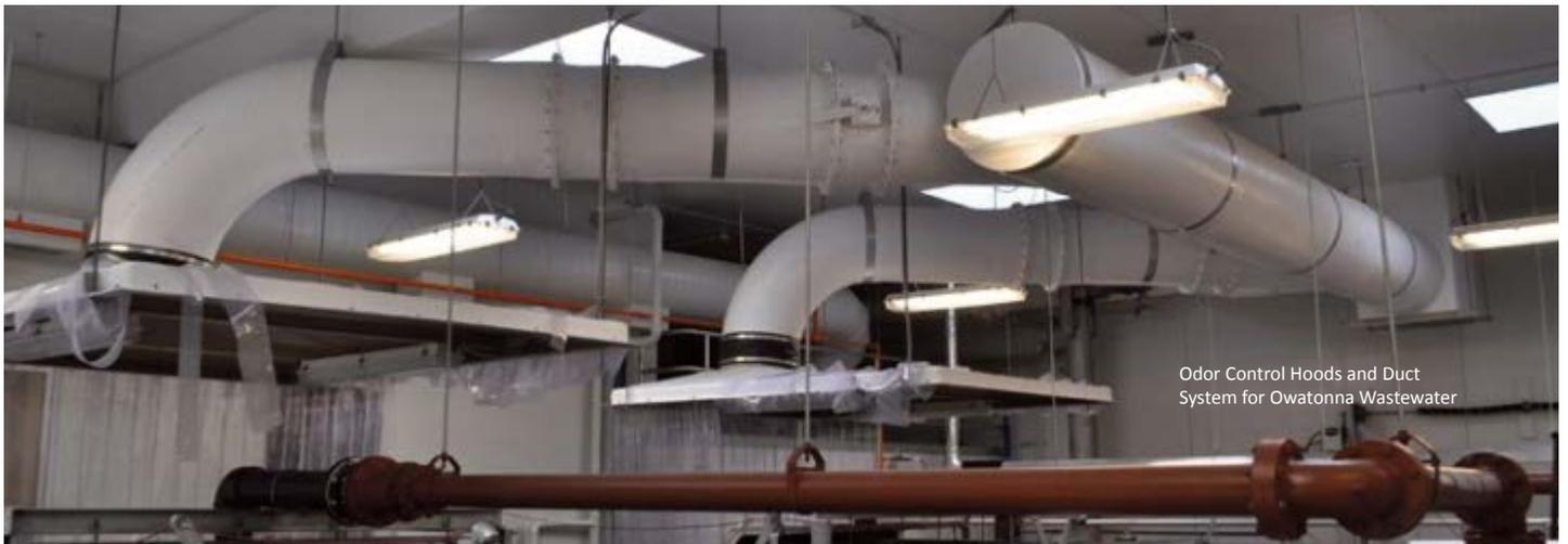
Odor Control Hoods and Duct System for Owatonna Wastewater
