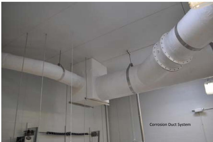
Corrosion Duct System
