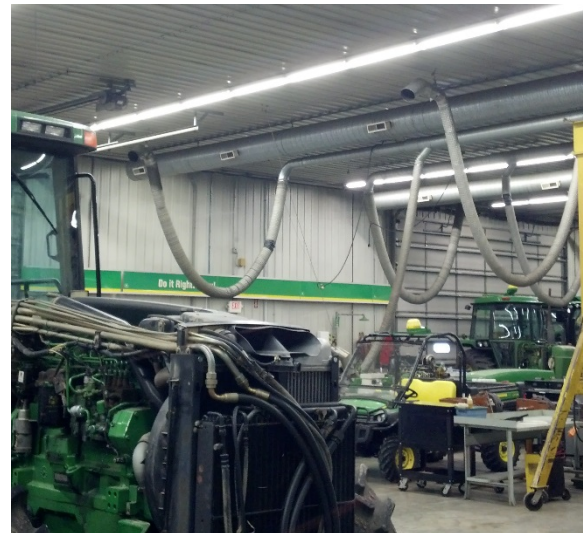
Existing Rope & Pulley System
