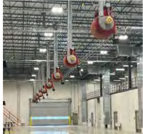
Motor Operated Hose Reel, with 4000 Series Exhaust Hose
